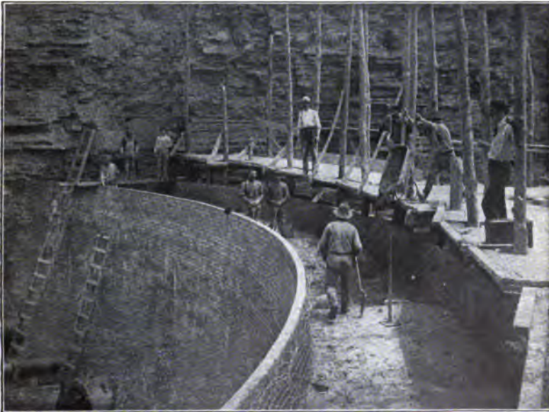
FIG. 2.—BUILDING THE SIX-MILE CREEK DAM.
